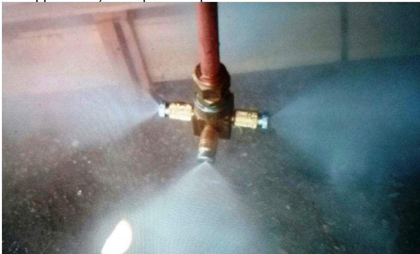
Photo 1: "GREEN UP FOG" spraying in a fuel tank
